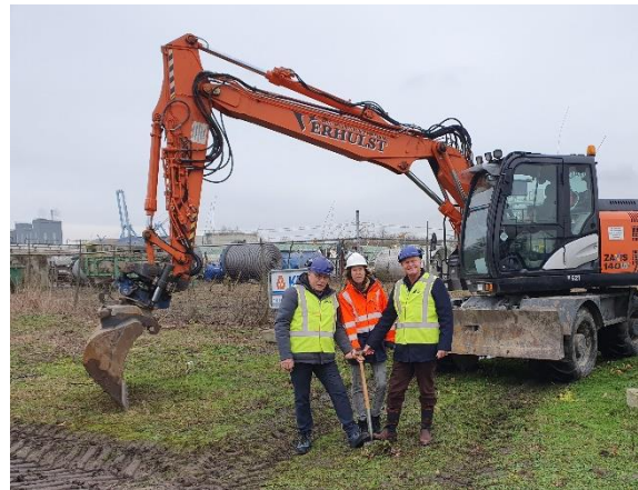
Figure 4: First spade in the ground on 16 December 2019 by Toine Janssen (Plant Manager PSLoop), Saskia Goole (Site-Manager ICL-IP), Lein Tange (Director PSLoop)
